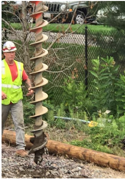
Wood Pole Installation
