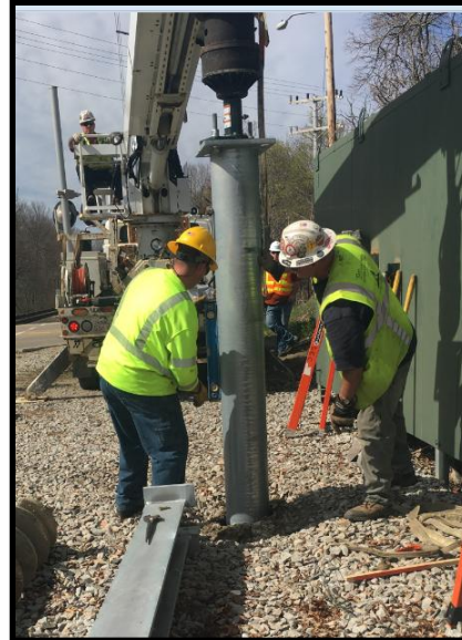
Antenna Base Installation
