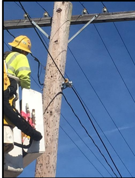
Overhead F.O. Installation
