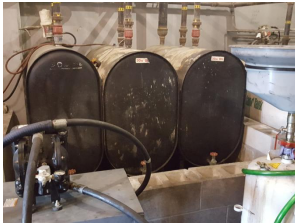
Oil Storage Tanks
