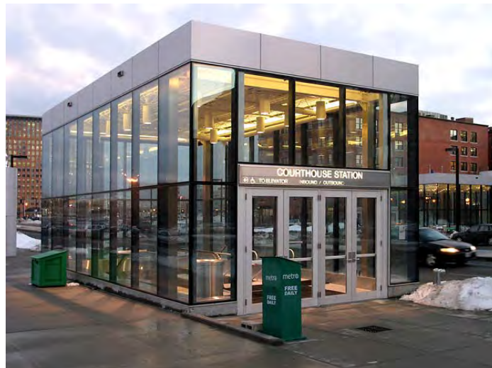
Courthouse Station (Silver Line)
