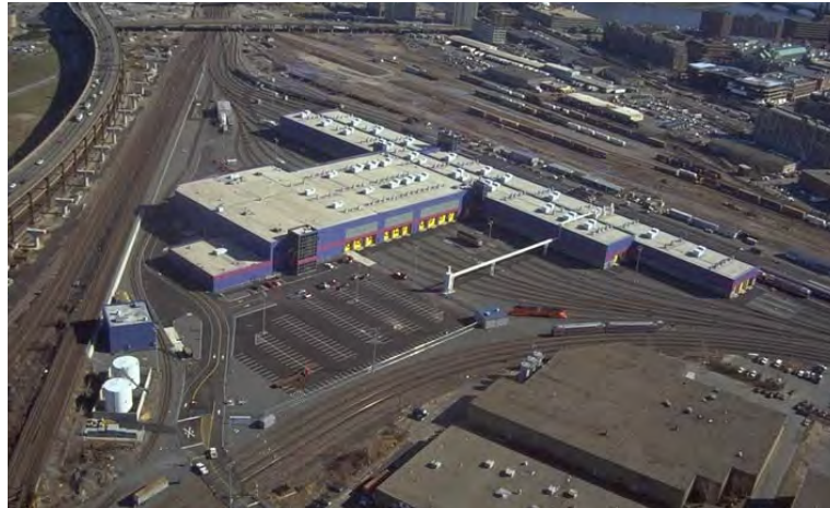
Boston Engine Terminal
